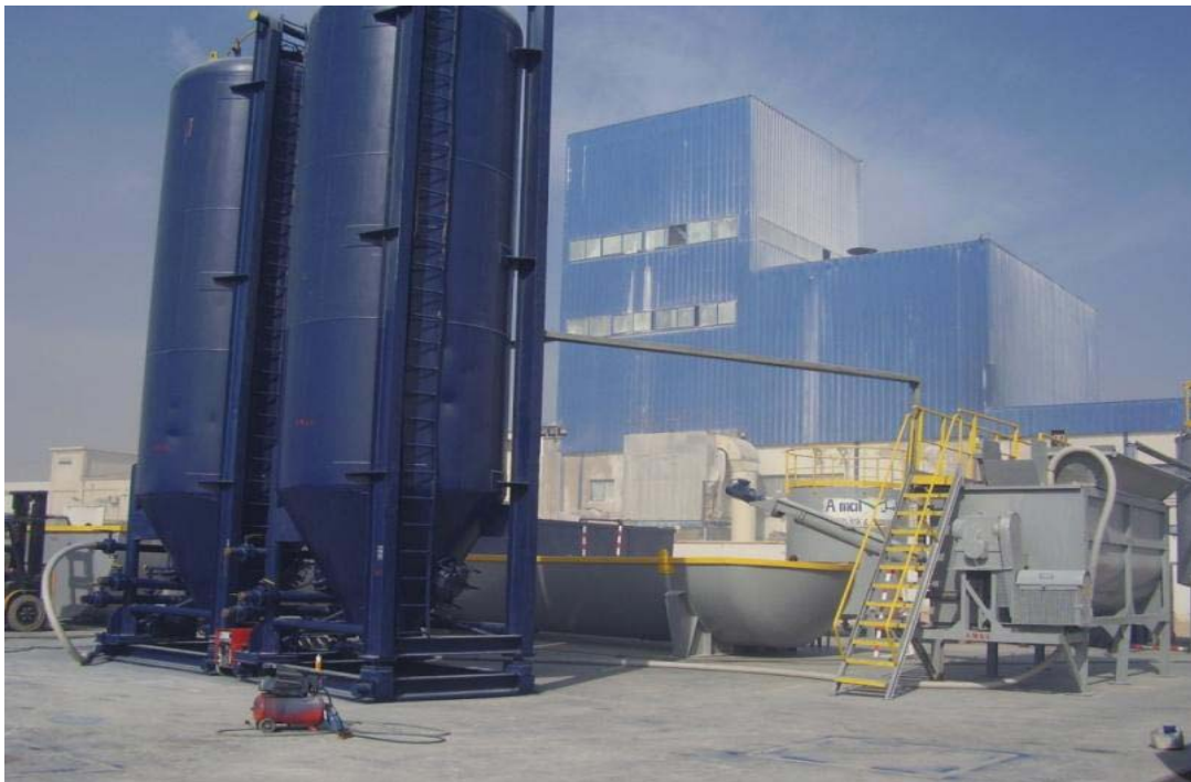
Drilling waste (mud /cutting) treatment unit
